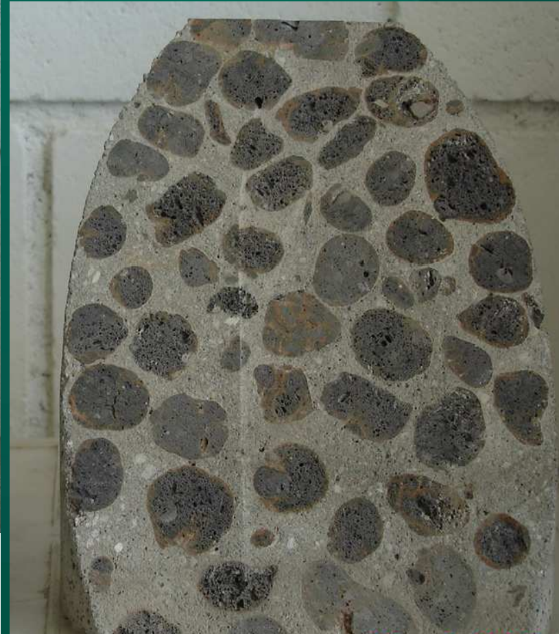
Concreto Leve com Argila Expandida
